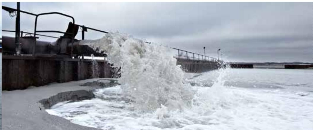
*Sand from navigation channels pumped from dredgers to drainage basins ashore*
