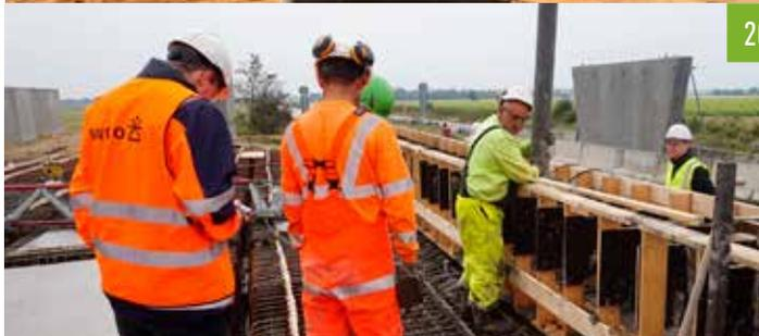
In 2017, the project took another important step when parts of two new demo bridges in Lolland were cast using green concrete. An important contribution to a full-scale view of the new technology.
